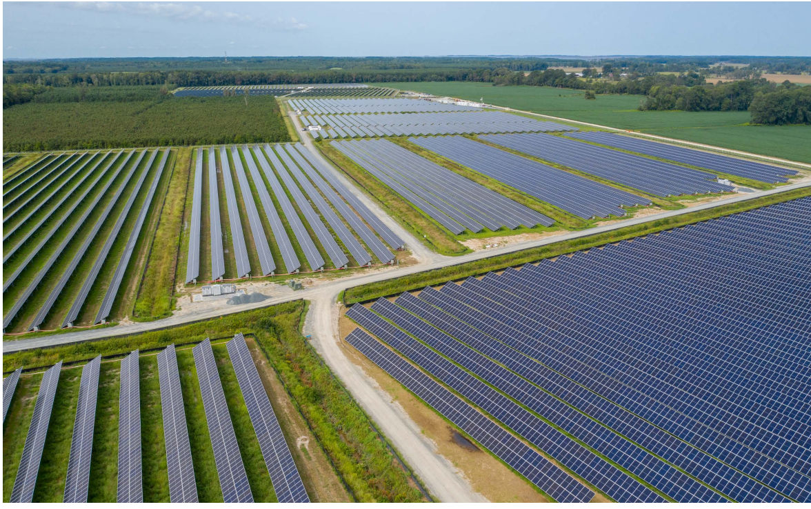
Altavista Solar (80 MW) Lynch Station, Virginia
